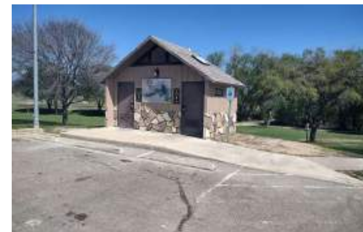
A small restroom installed in 2019 near the lakefront parking lot. The structure is pre-cast concrete, providing a durable and cost-effective solution to restroom needs.
