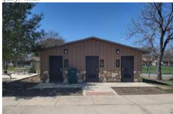
A new restroom was installed near the football field in 2020. The entrance road was also converted to one-way traffic around the building and the other driveway was blocked off to provide a safe spectator area.
